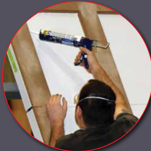
All joints are sealed with weather-proof caulking/sealant
